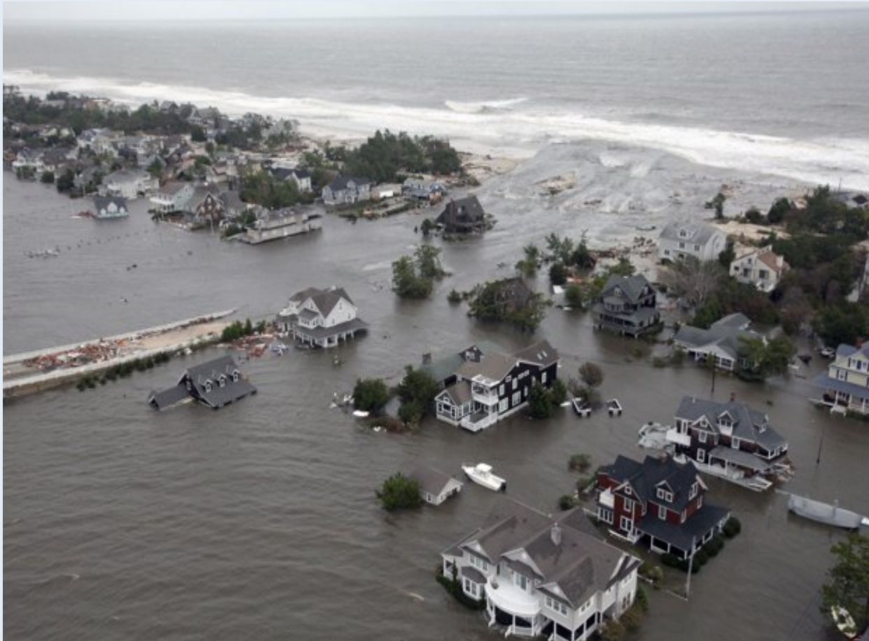
Hurricane Sandy coastal flooding in Mantoloking, N.J. Image Credit: New Jersey National Guard/Scott Anema.
